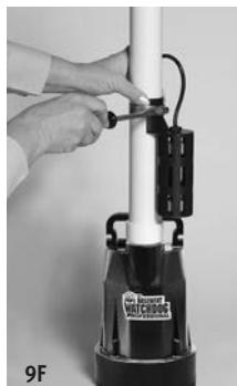
(Follow the instructions on the PVC cleaner and cement.) Then screw the new piece into the pump.
