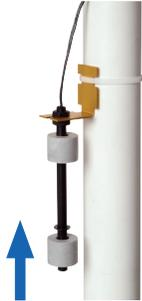
Lift the float up and let go. This will activate the pump. The control unit will run the pump for approximately 25 seconds so it can empty all the water in the sump pit. While the pump is active, water will come out of the  $\frac{3}{16}$ " hole that was drilled into the PVC discharge pipe. This is normal. The hole is needed to prevent an air lock within the system. **Do not** obstruct the hole or an air lock may prevent the system from activating.
