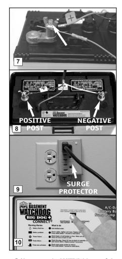
fluid sensor to the POSITIVE (+) post of the battery and slide the switch on the front of the controller to "Maintenance Free Battery"
