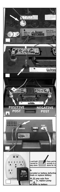
If you are not using the Basement Watchdog battery, you cannot use the battery fluid sensor. However, you must attach the sensor to the POSITIVE (+)
